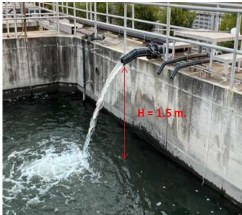
Figure 1 Cooling tower blowdown of a natural gas power plant in Phra Nakhon Si Ayutthaya Province, with a flow rate of 25,590 liters per hour .
