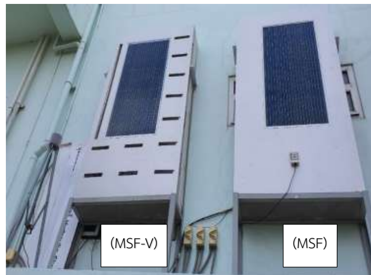
Figure 3 Installation of the Ventilated Multi-Purpose Modular Facade (MSF-V) and the Non-Ventilated Multi-Purpose Modular Facade (MSF)
