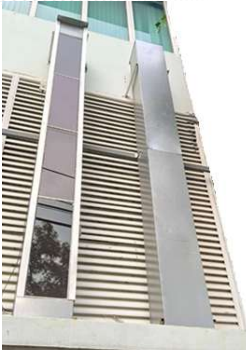
Figure 2 Solar chimney modeling and installation
